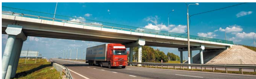
Autoroute M-4 Don
